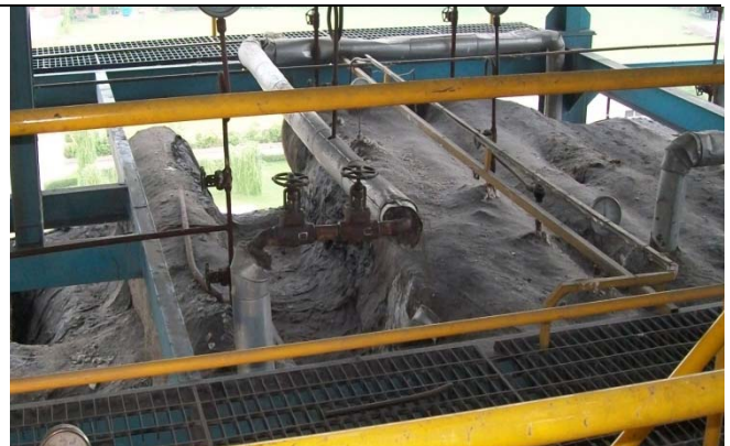
Photo 8: Sealing by POP helps to seal the roof easily.
