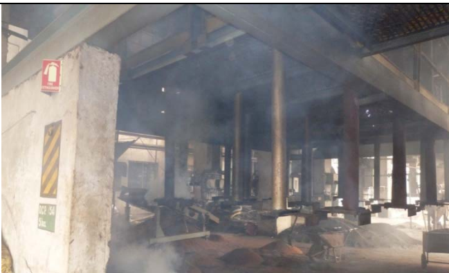
Photo 16- Smoke below airbox due to fire inside cross.
