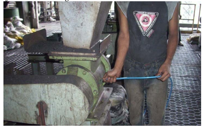
Photo 19: Arrangement to clean the feeder before it gets plugged.
