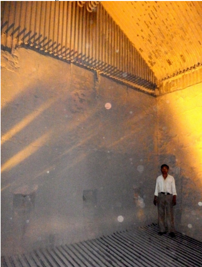
Photo 9: SA ports design needs improvement. They are placed close to radiant SH coils.
